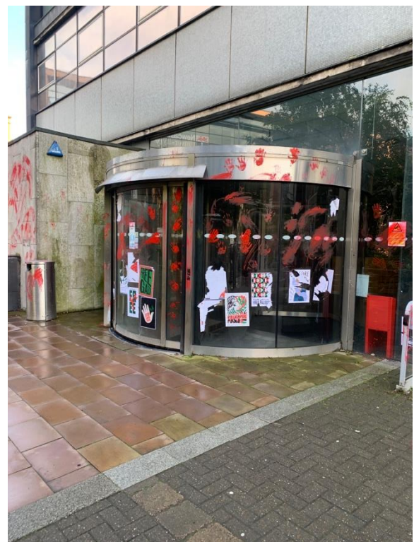
Below: 28/05/25, the Herschel Building following its redecoration in the night.
